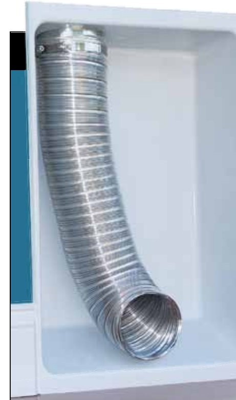
Unprotected Exhaust Hose is a Fire Hazard
