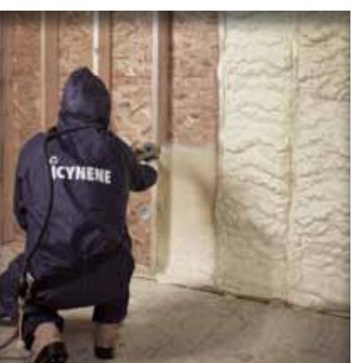
Though dense-pack cellulose and fiberglass batts offer decent R-values, they pale in comparison to liquid foam. Foam is sprayed into wall cavities and expands to fill cracks and crevices, creating a tight seal that minimizes air leakage. This high-performance product is popular with custom builders.
