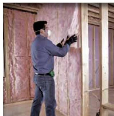
Traditionally, the overwhelming choice for production home builders has been batt insulation, which usually means fiberglass but also includes mineral wool.
