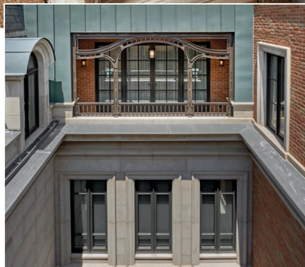
TOP: The dining room of the Lincoln Park Transitional Home offers a glimpse of the flowing staircase with its custom metal railing and continuous handrail. Interior and exterior custom steel-and-glass openings allow natural light to permeate the living spaces.
