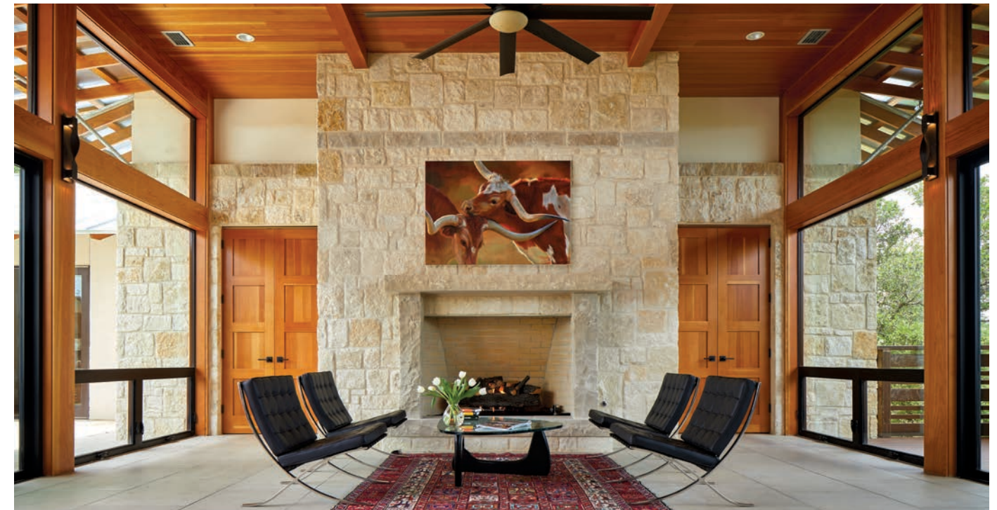
In the living room of Augusta, Lueders limestone on the walls and floors recall the workmanship of German immigrants who settled the region in the 19th century. The centerpiece is a shallow, Rumford-style fireplace that heats the large space during the winter months.
