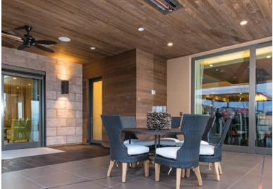
Nichiha's fiber-cement ArchitecturalBlock (top) creates a modern look with subtle seams. It is offered in Gray, Mocha, and Tuscan. Thermory's 1-by-4-inch tongue-and-groove ash siding (above) is sourced from sustainable forests and thermally modified to prevent mold and increase stability.
