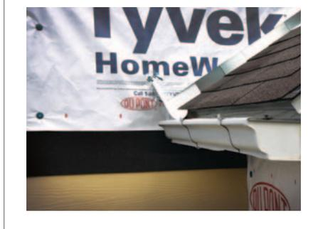
**Figure 4.** Torn housewrap admits water; untaped seams are leaks in the air barrier. Photo: Pacific Northwest National Lab
