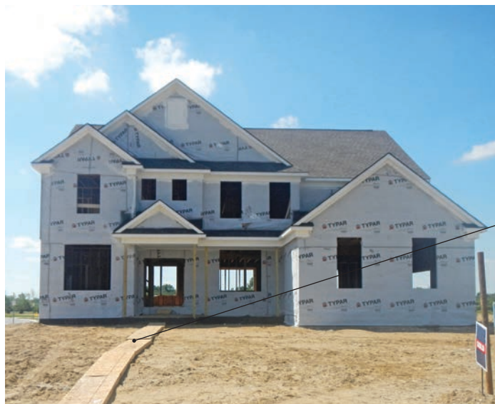
CLEAN INTERIOR SWEEPED AND STOCKED WITH DRYWALL STACKED FLAT
