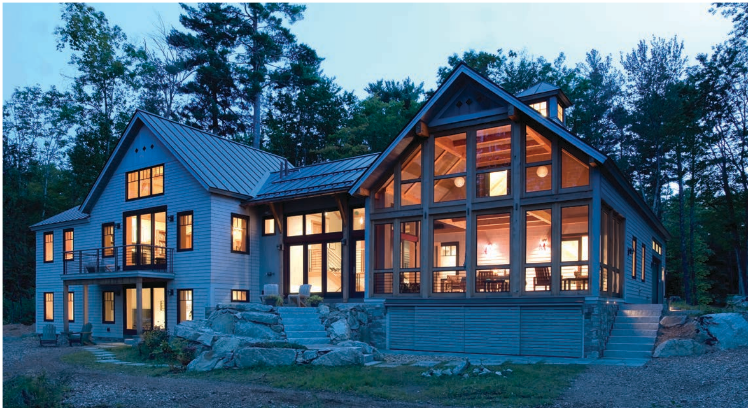
Fabricated by Bensonwood, this 3,063-square-foot custom home in New Hampshire includes a high-performance building shell, low-E windows, radiant-heat flooring, a heat recovery ventilation system, LED lighting, and many locally sourced materials.
