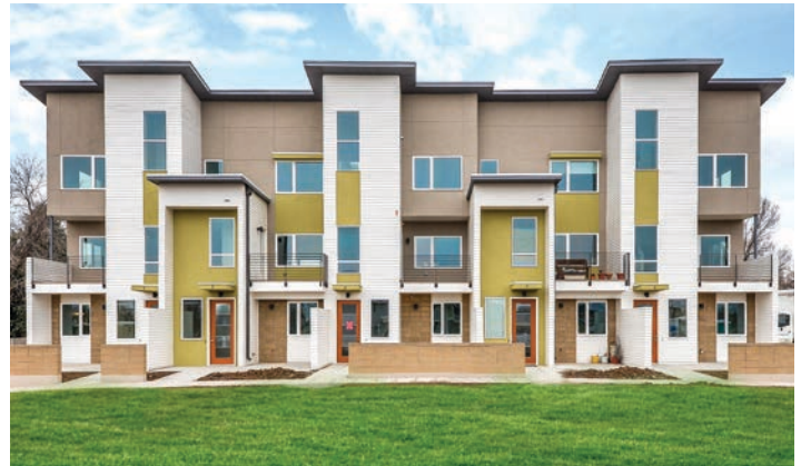
Revive, in Fort Collins, Colo., by Philgreen Construction and Revive Properties.
